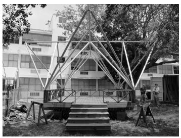
Figure 7. Framing and platform for Eco-tent with the canvas removed.
